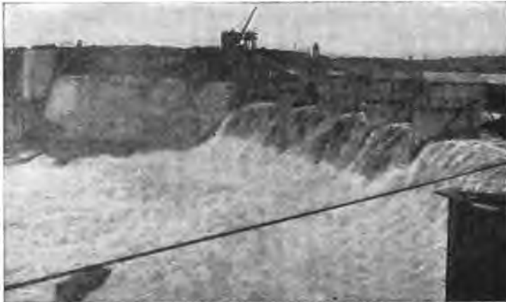
Spillway of Gatun Dam
